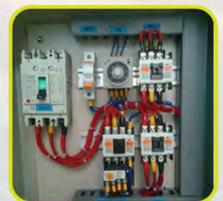
Star Delta Motor Starter
